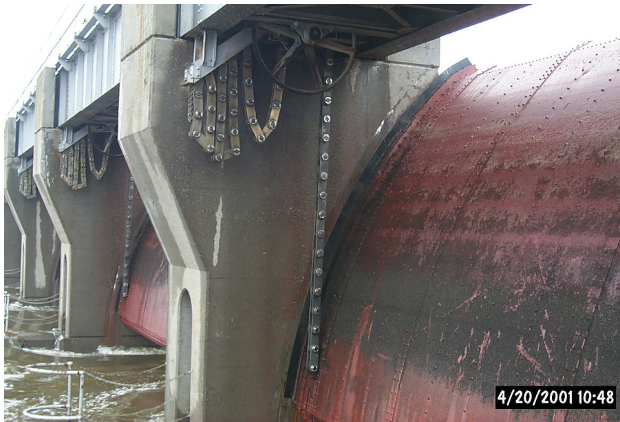
Figure 3-2. Typical Chain Installation
